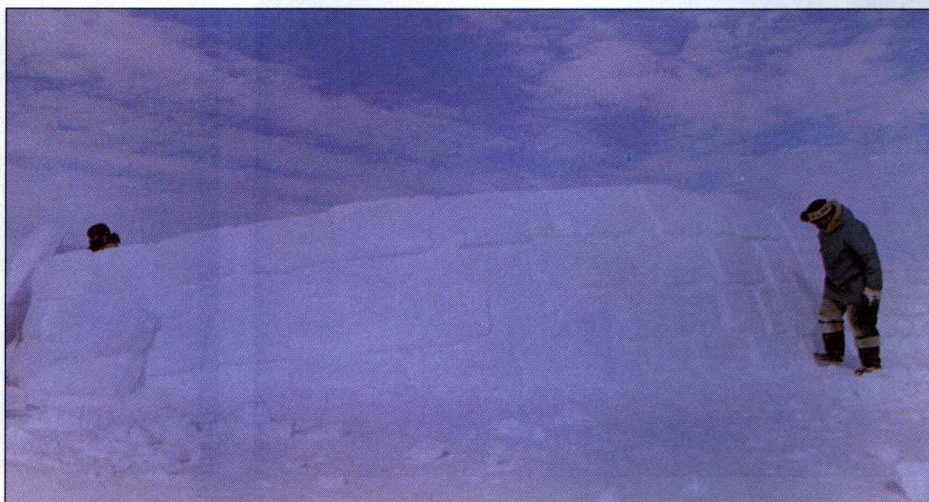
This is a qaggiq. Aipilik Inuksuk, left, piled, each snow block while other men, like David Irgaut, insulated the bottom.
